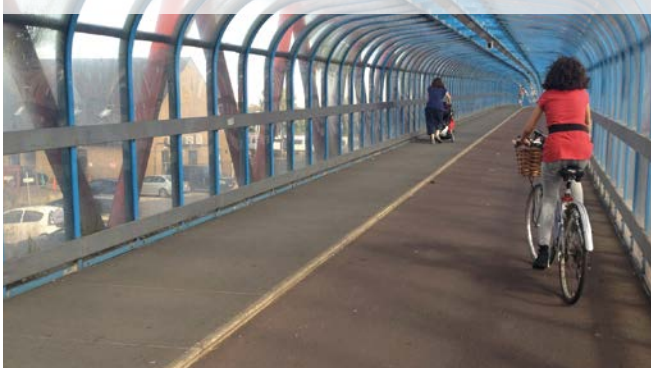
Figure 10.50: Covered pedestrian/cycle bridge across railway tracks, Cambridge
