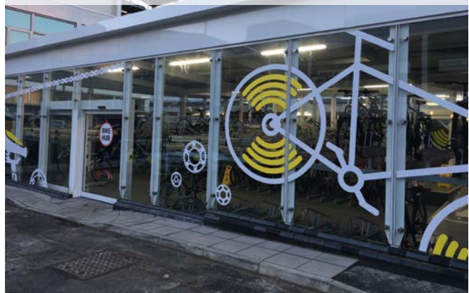
Figure 11.6: Secure cycle-hub (pass holders only) at Coventry station
