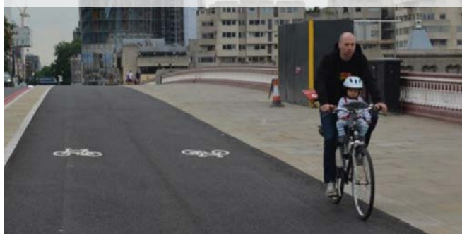
Figure 6.6: Footway-level cycle track with different surface materials to footway, London
