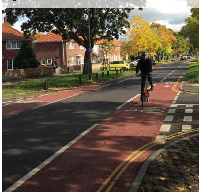
Figure 6.21: Centre line removal, Norwich
