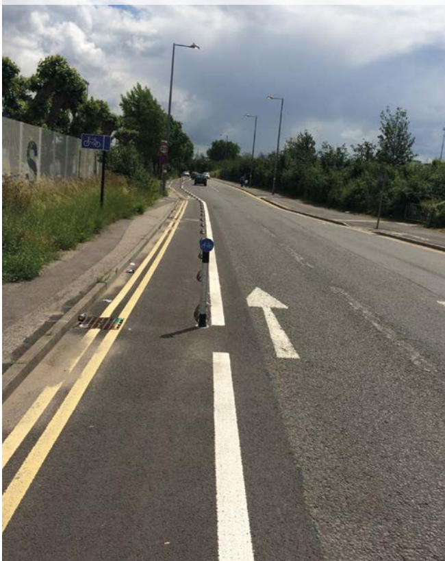
Figure 6.17: Low level light segregation features adjacent to a mandatory cycle lane
